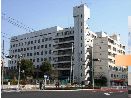
Building exterior before conversion
