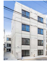
Reinforced concrete bearing wall structure, 4 Stories 1K : 11Units, 2DK : 1Unit, 2LDK : 1Unit
