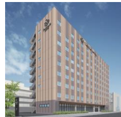
Image of Building Exterior
