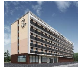
Image of Building Exterior
