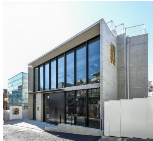
Newly built, steel-reinforced concrete structure with flat roof, 2 stories
