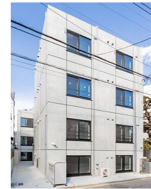
Reinforced concrete bearing wall structure, 4 Stories 1K : 11Units, 2DK : 1Unit, 2LDK : 1Unit
