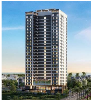
Reinforced concrete structure, 25 Stories with 2 basement floor 1LDK: 22Units, 2LDK: 176Units, 3LDK: 4Units
