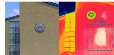
Infrared rays can identify floating tiles
