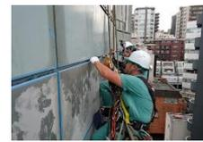
Checking for external Leaks also
