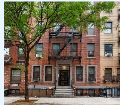
Value-up building appearance
