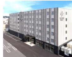
Tabino Hotel Kurashiki Mizushima Opened in February 2020, currently in operation
