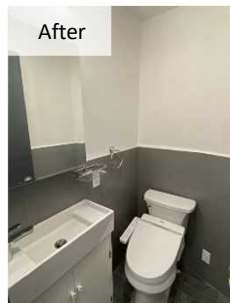
Separate bathrooms and toilets Installation of washlet toilets
