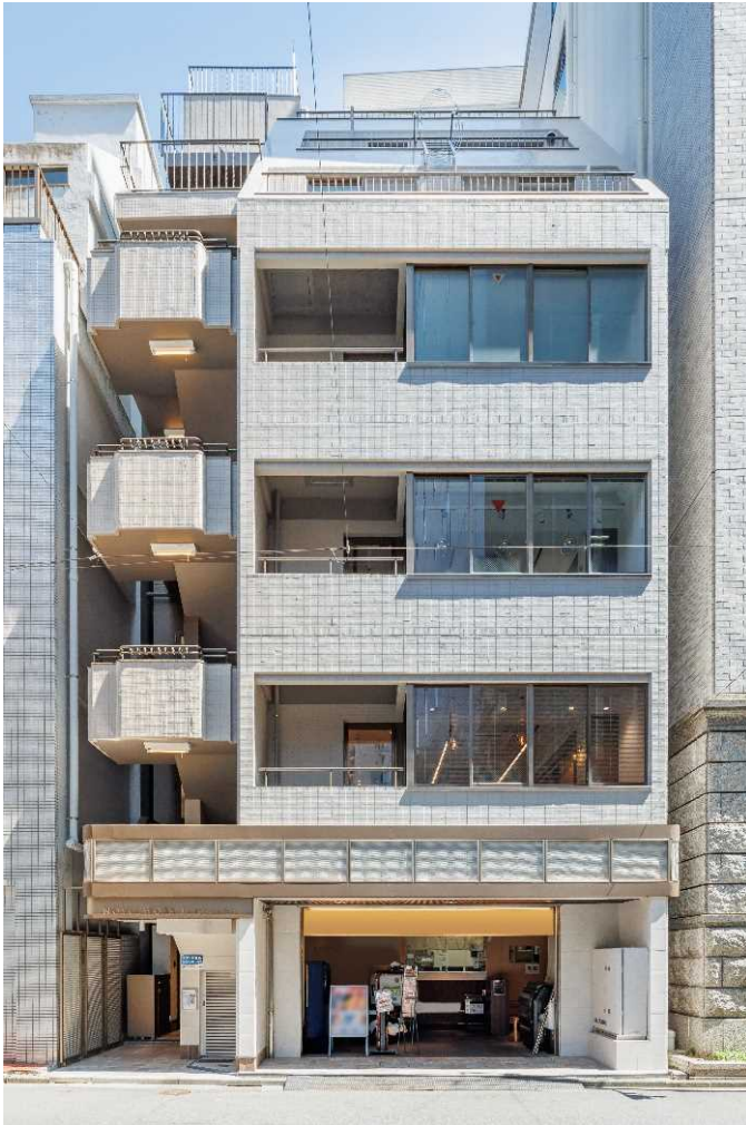
[Building exterior (after Replanning)] Kandajinbocho, Chiyoda-ku, Tokyo 7-story steel reinforced concrete and reinforced concrete building with deck roof
