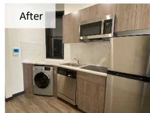
Installation of a built-in kitchen
