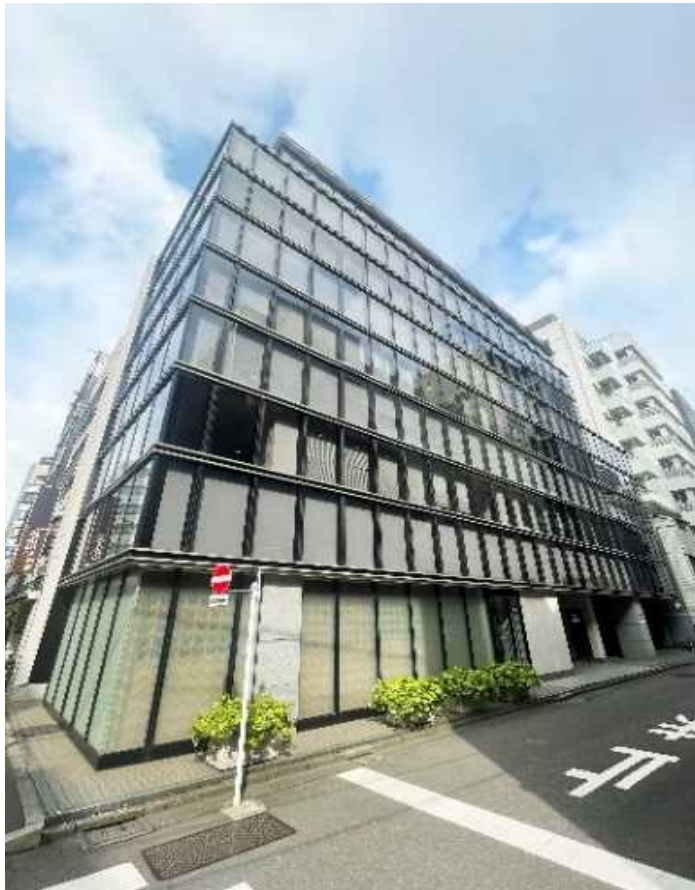
[Building exterior (after Replanning)] Kandasudacho, Chiyoda-ku, Tokyo Steel-framed and steel reinforced concrete structure with deck roof, 8-story building with 1 basement
